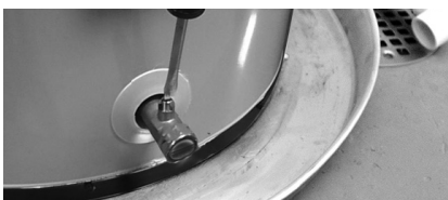
Figure 42 - Draining the water heater.
