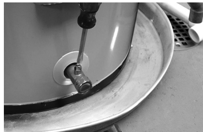
Figure 20 - Draining the old water heater.
